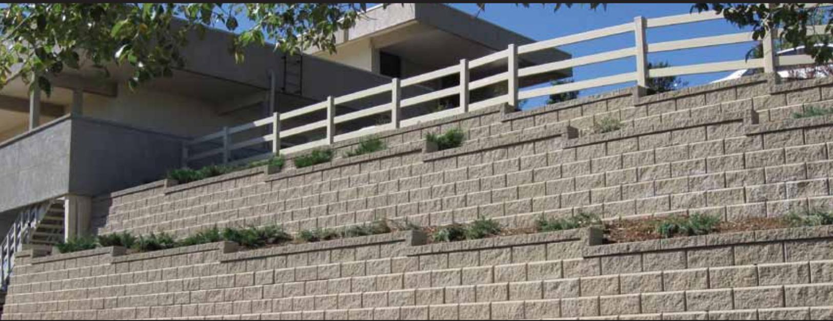
**Keystone Victorian Stone™** is made of high-strength, low absorption concrete for long lasting structures. All structural units are interconnected using high-strength fiberglass pins for strong shear connection. The connecting pins allow for ease-of-unit alignment and a secure positive mechanical connection with soil reinforcement materials. Keystone's patented fiberglass pin system is the critical difference providing the safety and security of a structural retaining wall solution!
